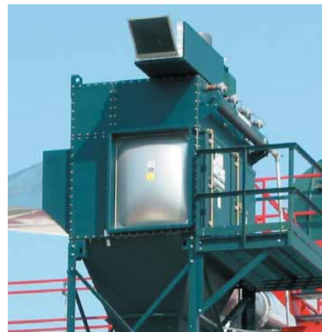
Explosion Vent—NFPA Rupture Panel
